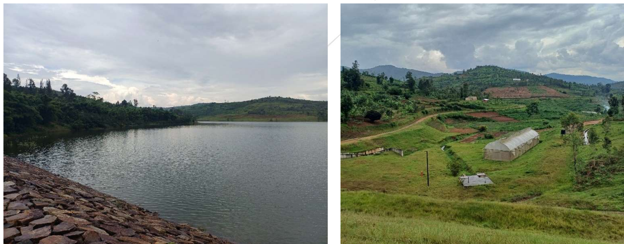
Figure 9-4: Nyanza Hillside Irrigation Dam (left) and irrigated land and canals (right)
