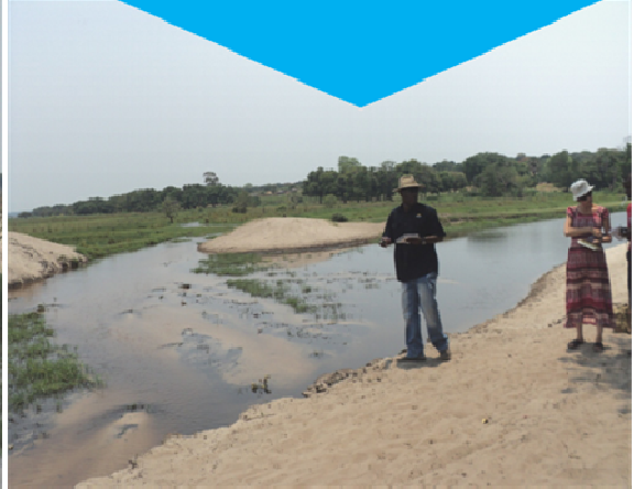
Muoyowamo Canal at the entrance of the upper Musiamo canal – see sand deposits!
