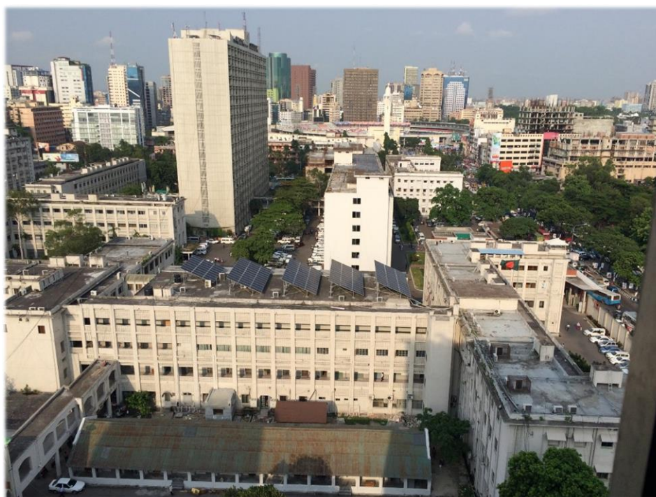
50 kWp rooftop solar PV installation on Secretariat building in Dhaka.
