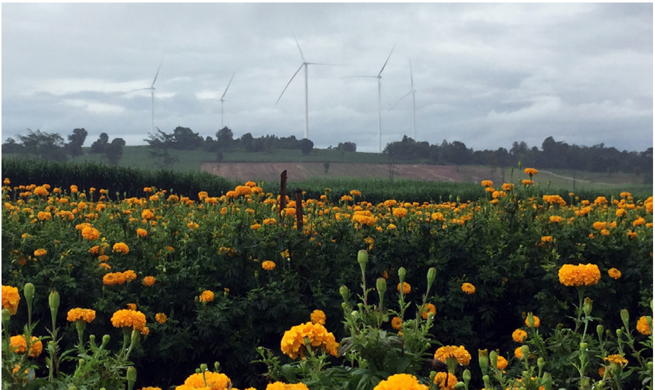
Theppana Wind Farm, Thailand
