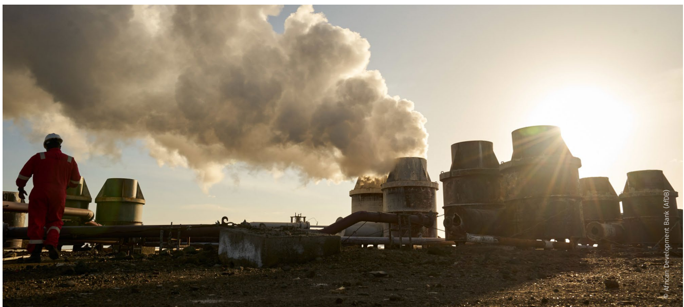
Menengai Geothermal Development Project, Kenya.
