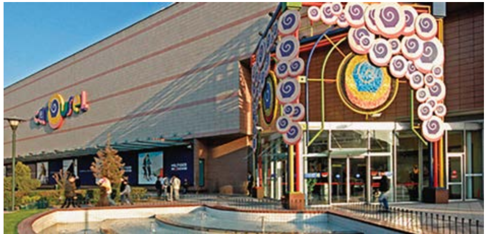
The Baymer Tourism and Investment Company, owner of the Carousel Mall in Istanbul, Turkey, invested in a number of energy efficiency measures financed through Vakifbank with $2.6 million from EBRD’s TURSEFF and the CTF. The company expects to reduce annual energy costs by $484,000 and cut greenhouse gas emissions by over 2,000 tons of CO 2 equivalent.
