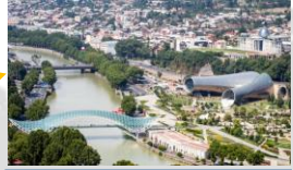
Georgia Energy Storage
