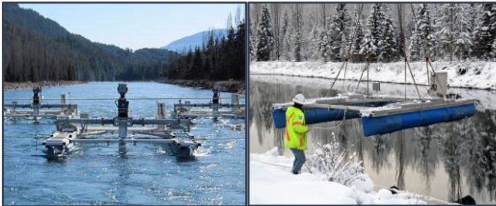
Figure 4.5: Floating Micro-Hydro Systems
